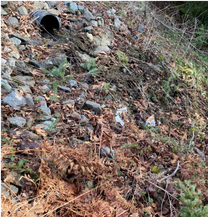
Photograph 9. Culvert 2 outfall with splash pad at station 40+50.
