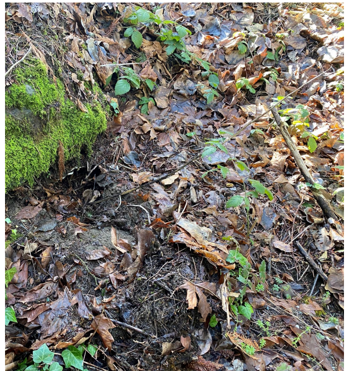
Photograph 4. Existing southern inlet to the existing detention pond at station 15+25.
