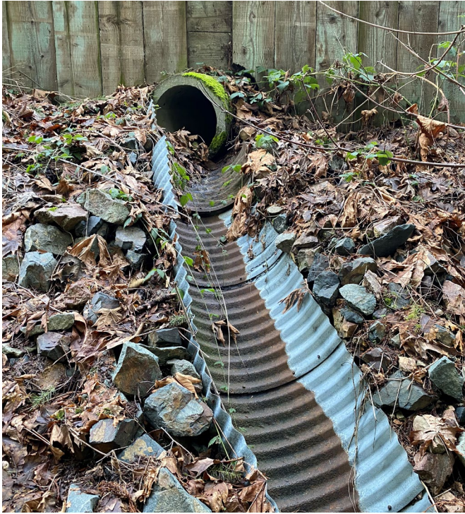
Photograph 9. Culvert 2 outfall with splash pad at station 40+50.
