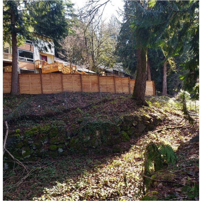
Photograph 2. Existing detention pond at station 15+25 looking south from the riser structure.
