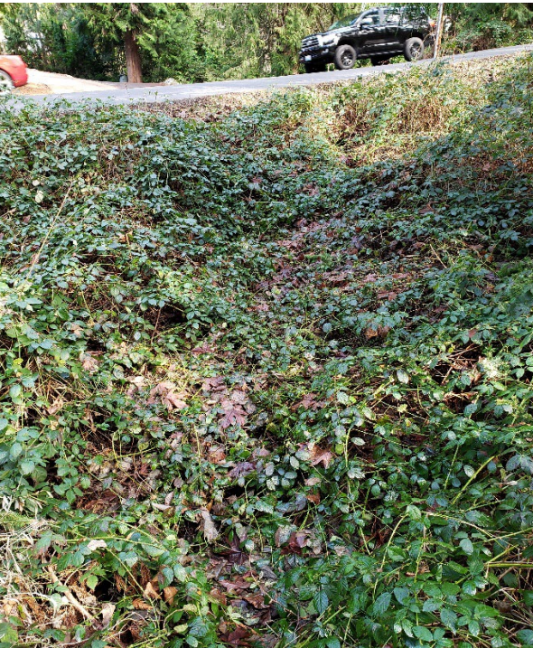
Photograph 7. Vegetated area at the outfall of culvert 4 at station 31+50.
