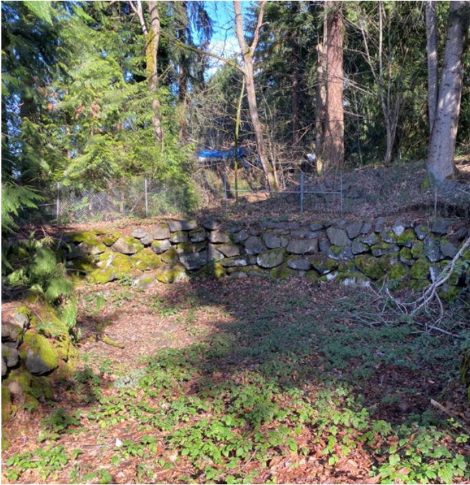
Photograph 1. Existing detention pond at station 15+25 looking north from the access ramp.
