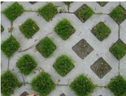
Figure 47. Grass pavers, Bainbridge Island, WA.
