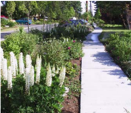
Figure 46. SEASStreet vegetated bioretention swale. Seattle, WA.
