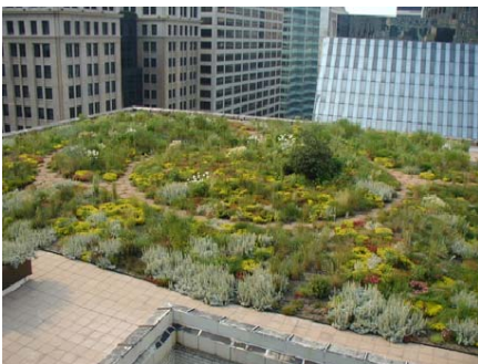
Figure 48. Green roof, Chicago, IL.
