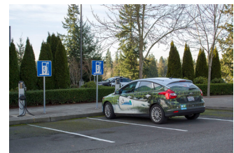
Electric vehicle charging station at City Hall
