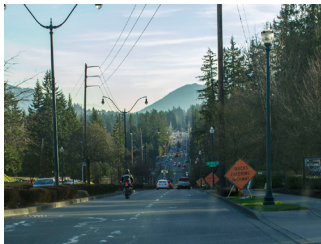
Construction on 228th Ave SE
