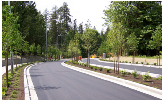
Construction on Pine Lake Transit Access Road
