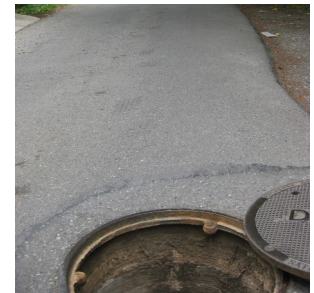
Manhole with cover removed
