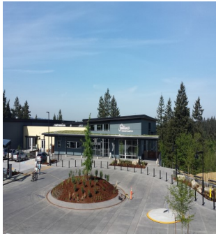
Sammamish Community and Aquatic Center green roof
