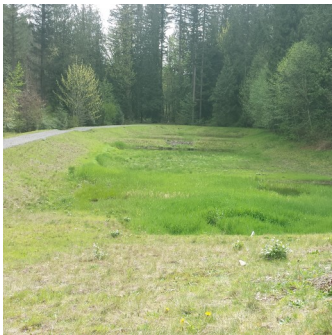
244th Avenue NE stormwater facility
