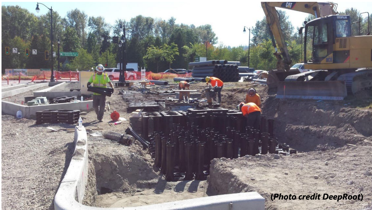
Figure 5. Bothell downtown core Silva Cell installation – Before
