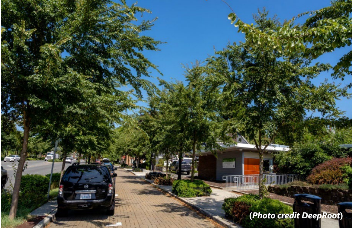
Figure 6. Bothell downtown core Silva Cell installation – After
