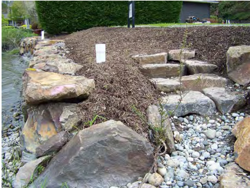
Photo 1: Revised maximum 60-foot long bulkhead to remain.
