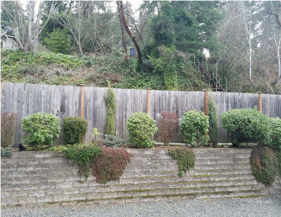
Image # 3 Concrete Block Wall with 6 ft. Cedar Fence
