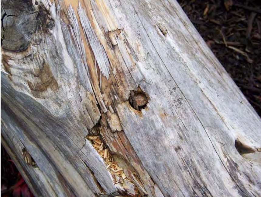
Photo 3: Rebar stake through log along buffer boundary.
