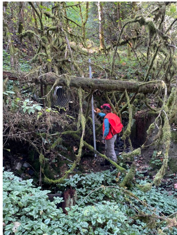
Photo 53. Perched culverts conveying Kanim Creek at SE 19th Street, STA 3800 (September 2023).
