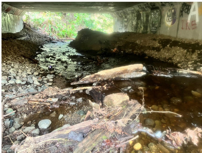
Photo 6. Looking downstream under 210th Place SE bridge, STA 8450 (March 2023). Notice the mound of sediment next to right wall at the downstream end of the bridge.
