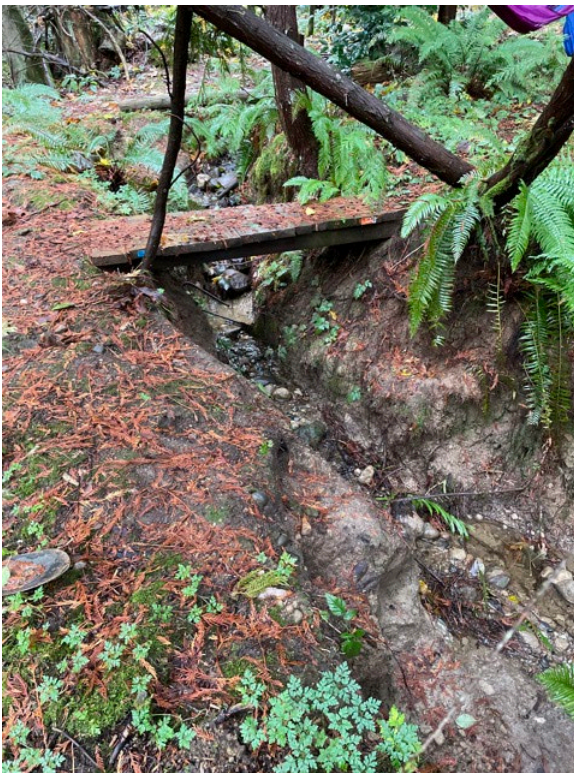
Photo 52. Channel formed downstream of stormwater outfall from Stormwater Facility D92924.
