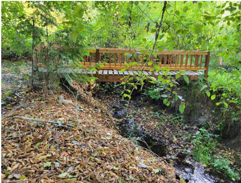
Photo 28. Small wooden pedestrian bridge over Pine Lake Creek in the lower residential reach, facing upstream, near STA 2260. Note channel incision and lack of vegetation (September 2023).
