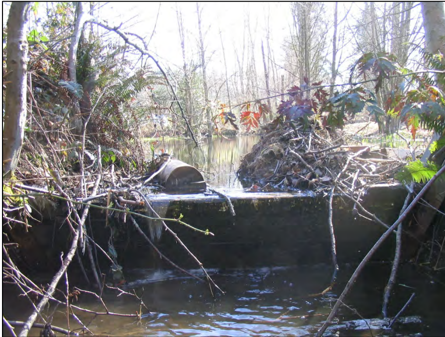
Figure 15. Pine Lake Outlet Weir
