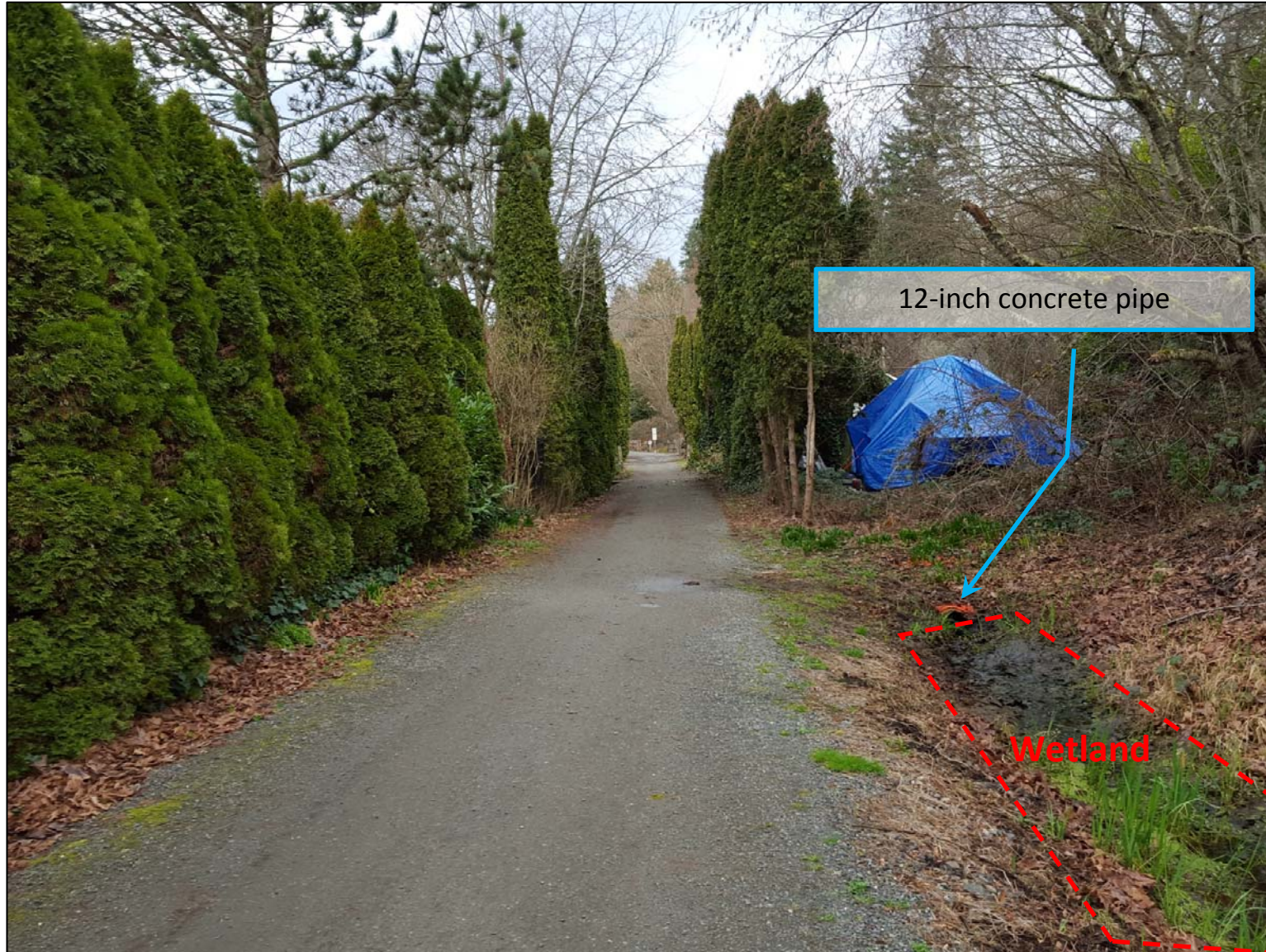
Picture 1 – This 12-inch pipe was viewed with a pipe camera. This pipe is shown in orange spray paint and connects to the Wetland at this location. (Looking north)
