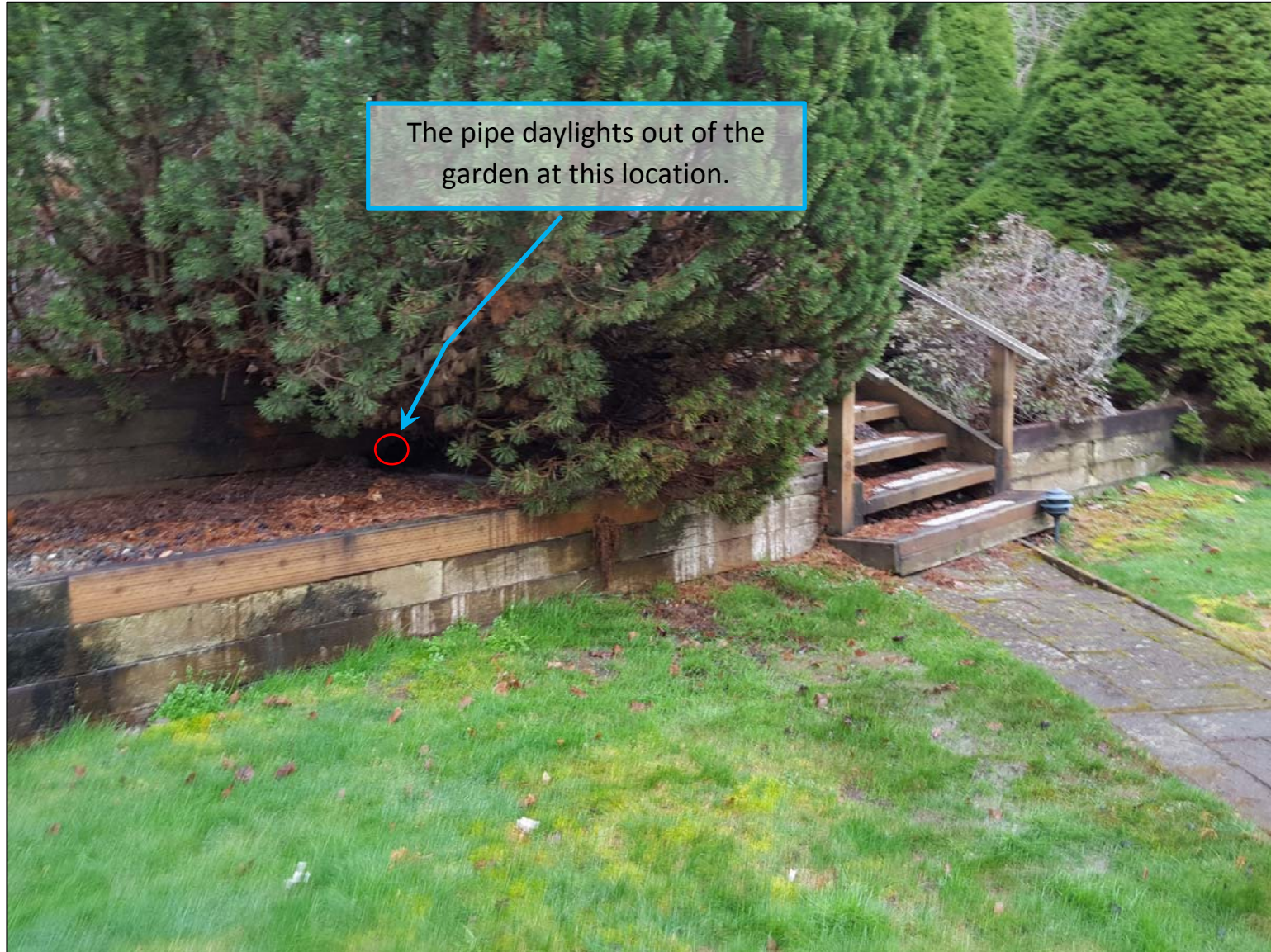
Picture 4 – Approximately 20' feet from the 90 degree bend on the east side of the trail, the pipe daylights out of the wood garden wall at 833 East Lake Sammamish Parkway NE. (Looking southeast)
