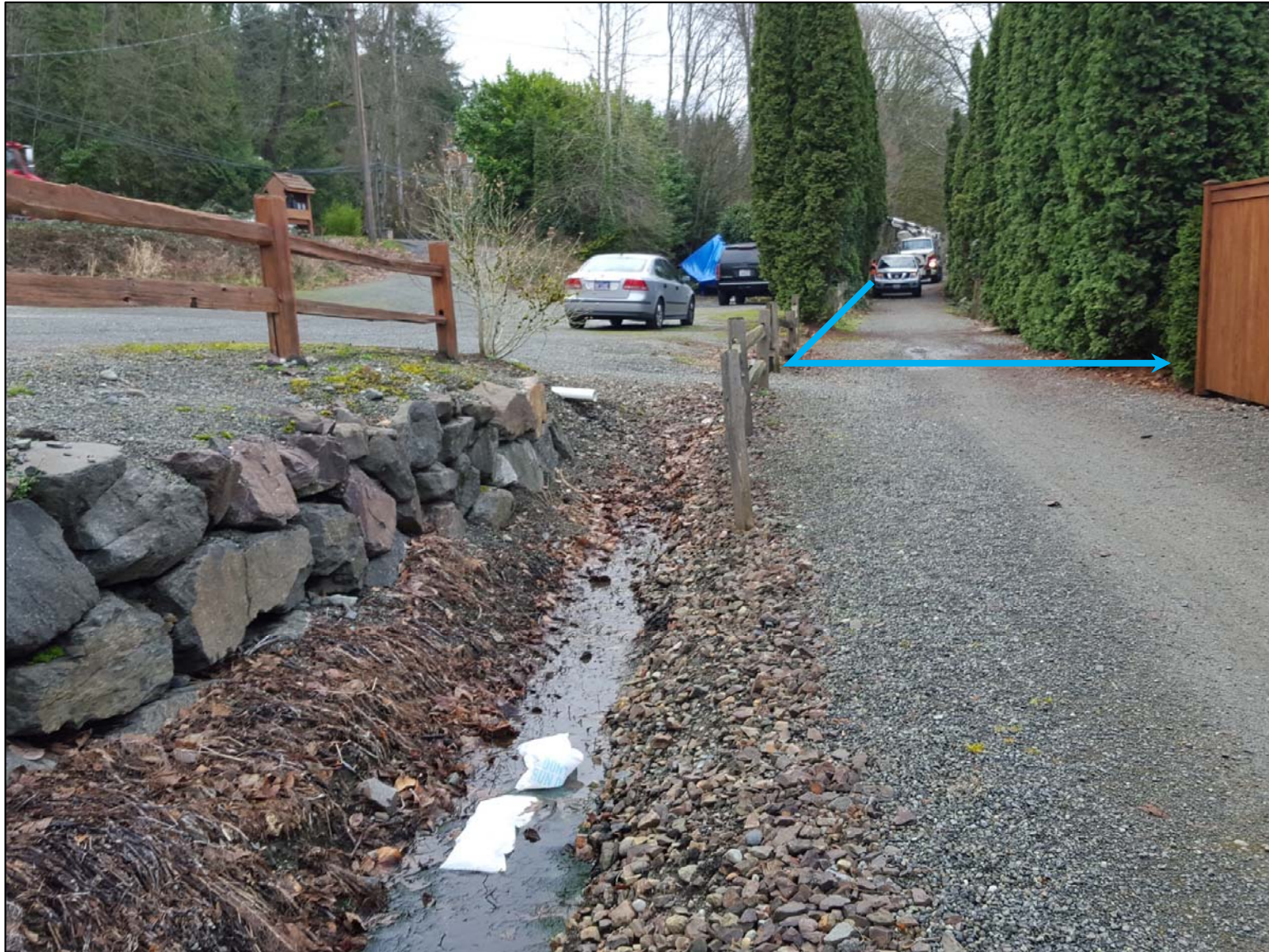
Picture 3 – Looking south towards the drainage line from Picture 1 and 2 (shown as blue line). The line takes a sudden 90 degree turn towards the lake. This picture was taken approximately 250 feet north of the beginning of the 12-inch concrete pipe from Picture 1. (Looking south)
