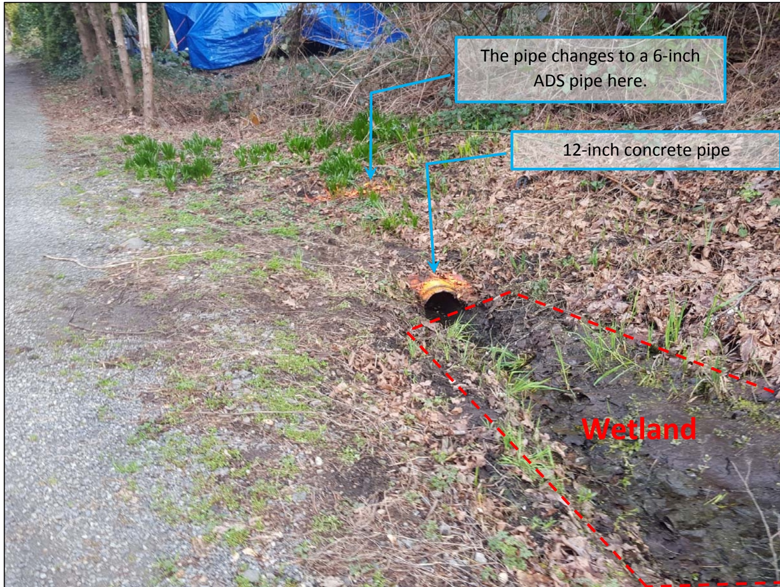
Picture 2 - The pipe changes from a 12-inch concrete pipe to a 6-inch ADS pipe. (Looking downward and northeast)
